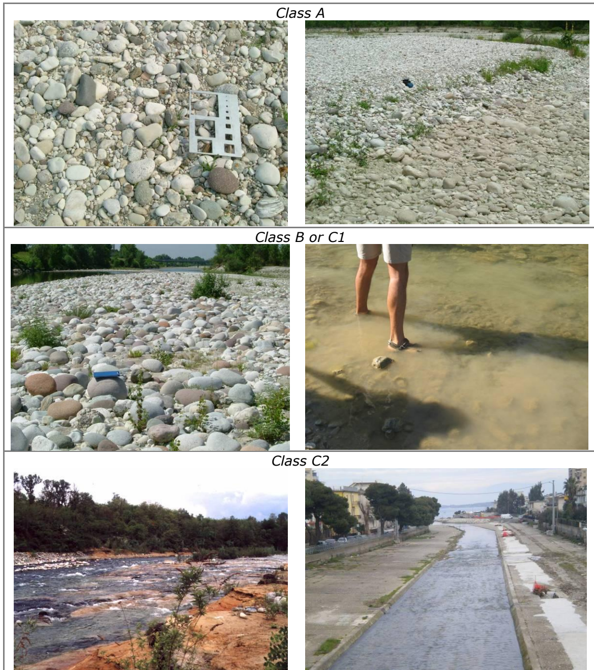
Figure 36 Alterations of substrate in partly- and unconfined channels. Class A : natural sediment heterogeneity in an unconfined channel. Class B or C1 : presence of armouring (photo on left) or clogging (photo on right) (assignment to Class B or C1 will depend on the extension of armouring and/or clogging along the reach). Class C2 : bedrock outcroppings due to bed incision (photo on left) or completely altered substrate because of bed revetment (photo on right).
