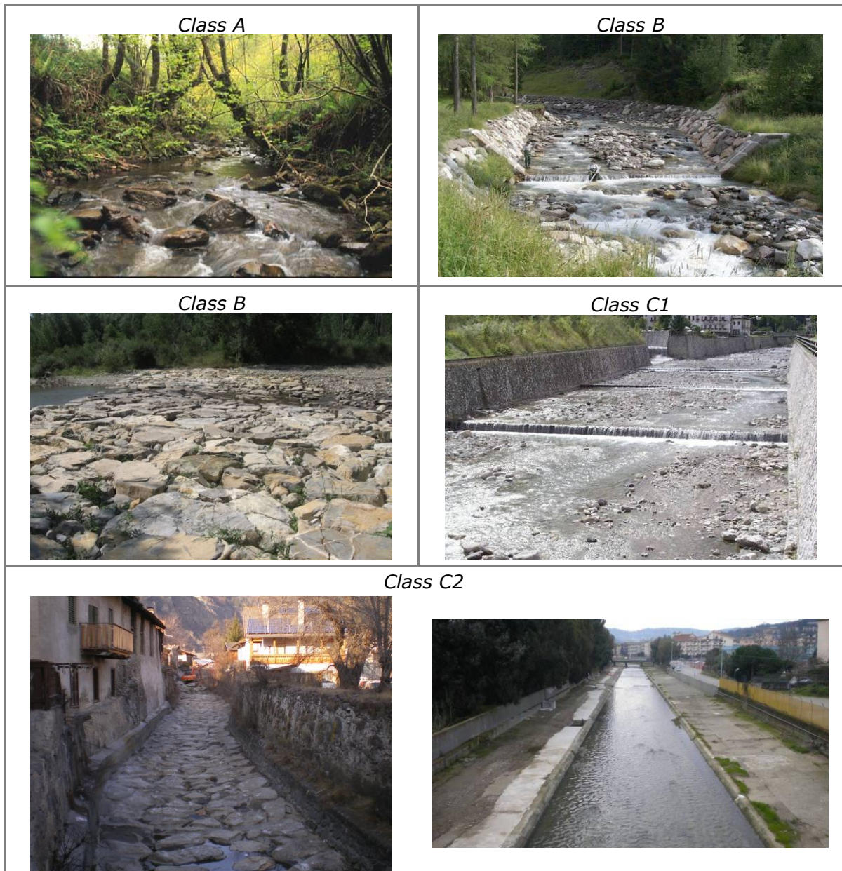
Figure 66 Other bed stabilization structures and revetments. Class A : total absence of other bed stabilization structures or revetments. Class B : presence of sills (first row on right) or mass ramps (second row on left) with low density. Class C1 : various sills and partial bed revetment. Class C2 : total bed revetment with impermeable systems.
